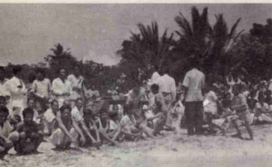
Piling up the sand for the foundation of the church at Barus Atjeh, Sumatra, so place will not be flooded when the heavy rains come.
